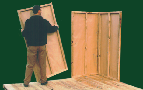
Shed assembly; wall panels
